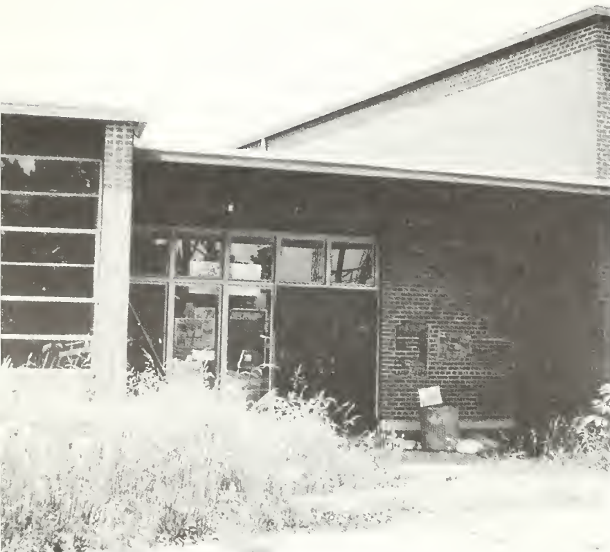
Before...an abandoned school.
